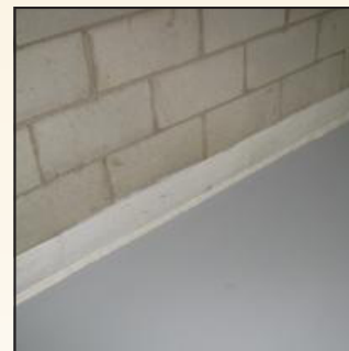
Urethane Perimeter Concrete
